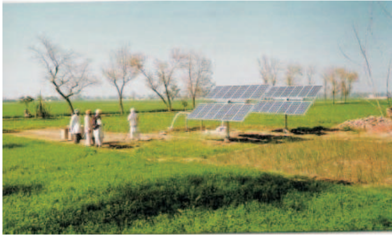
Figure 12.6 Photovoltaic Water Pumping
