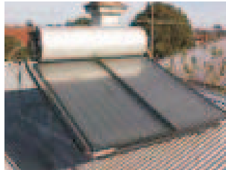
Figure 12.1 Solar Flat plate collector
